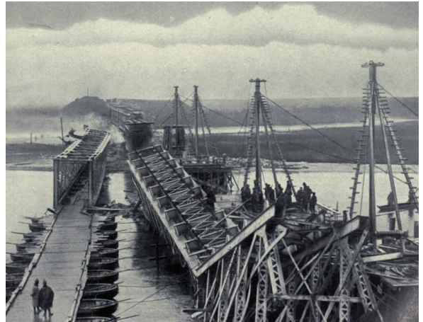
Rebuilding a destroyed railroad bridge on the Warta River. Source: www.gwpda.org/photos
